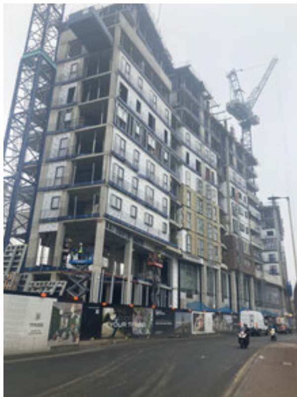
Plate 22: New Student Accommodation on the east side of Ilderton Road
