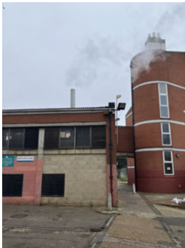
Plate 76: Connection at the Cossall Estate Boiler House
