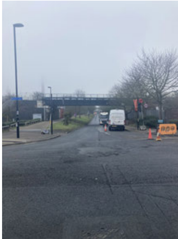
Plate 9: Surrey Canal Road looking East from the junction with Ilderton Road, the current ground surface falls away to the east, as the historic canal was bridged at this point.
