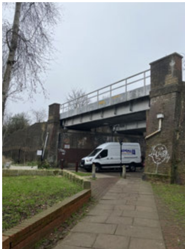
Plate 78: View to the Railway Bridge outside the Boiler House, looking Southeast
