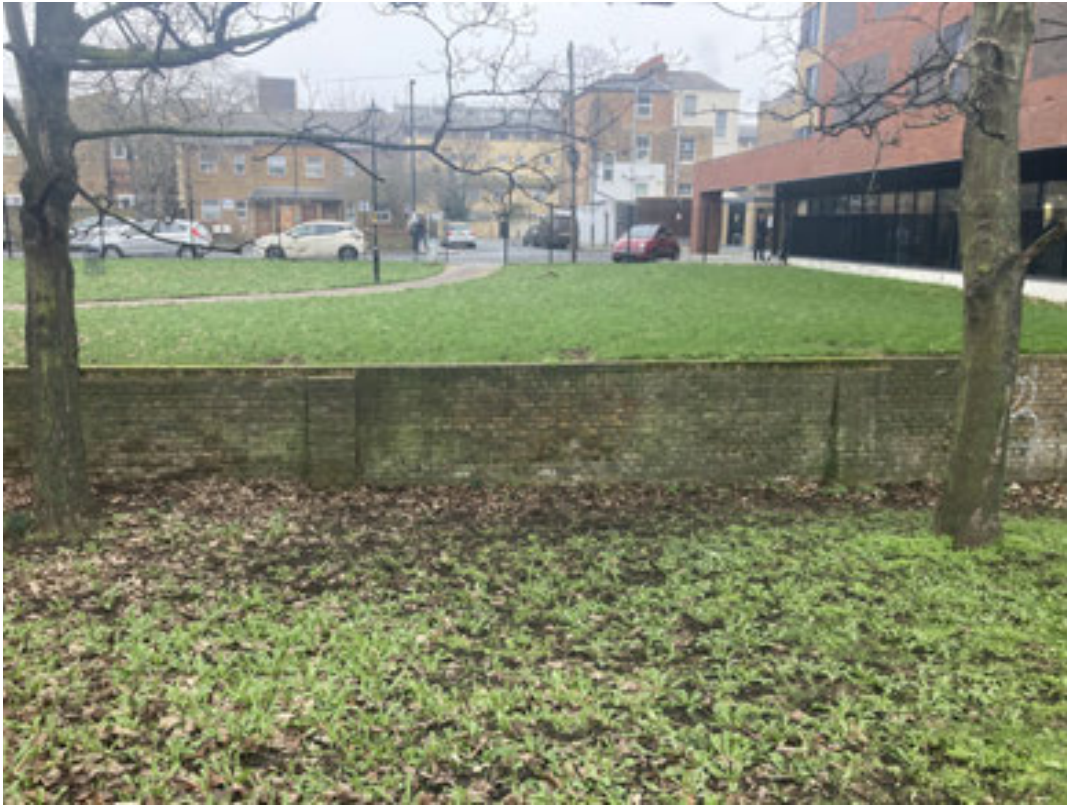
Plate 63: Looking East from Surrey Canal Walk to the change in height on Bonar Street at the historic location of Eagle Wharf beside the Grand Surrey Canal, The wall may be original architecture surviving from the canal.
